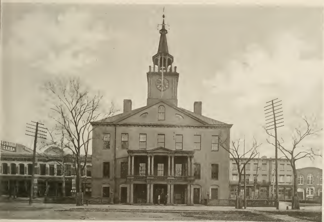
CITY EXCHANGE AND BAY STREET.
